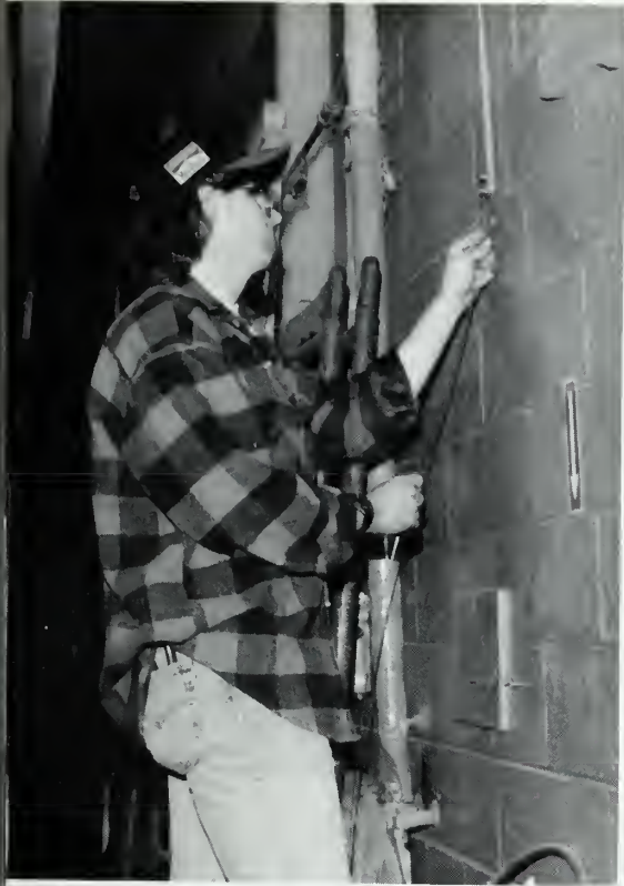
Electrical Peter Donahue
